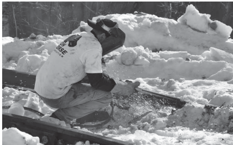
Iron Horse worker removing rails in Massachusetts
