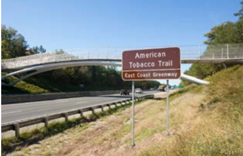
Top: Signage for bike/pedestrian bridge over I-40 in Durham, North Carolina.
