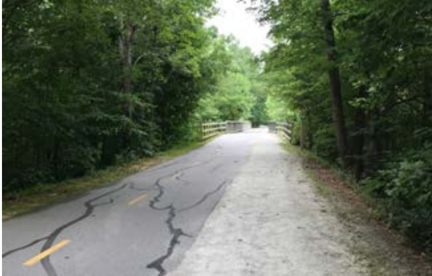
A portion of the American Tobacco Trail in Wake County, N.C., features an asphalt trail with stone-dust shoulder alongside it.
