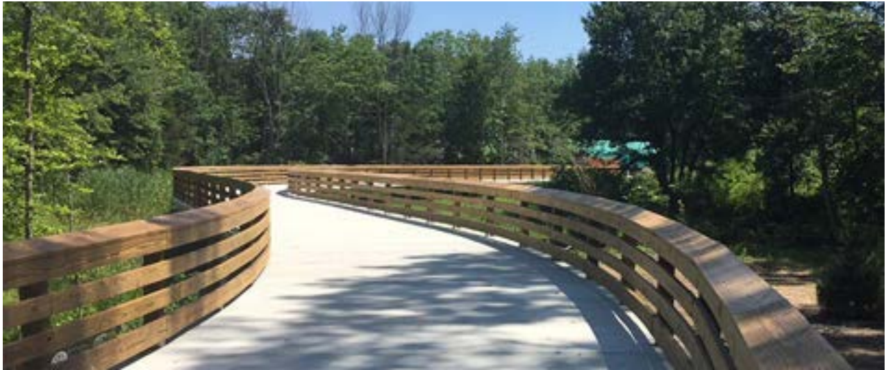
Permatrak concrete surface on boardwalk along Farmington Canal Heritage Trail, Cheshire, Connecticut
