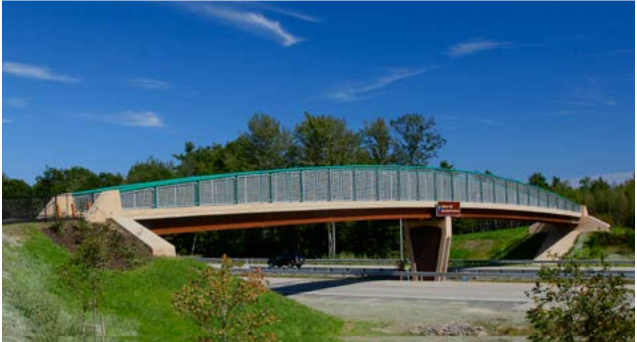
Eastern Trail's John R. Andrews Bridge over the Maine Turnpike
